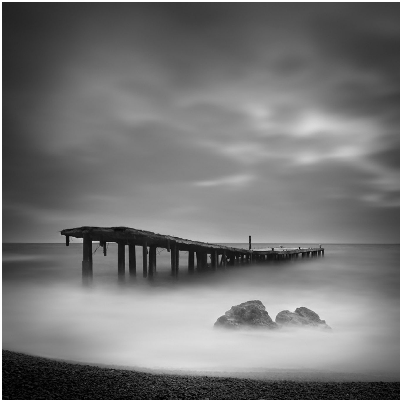
Destroyed pier , Автор: Yury Bird
